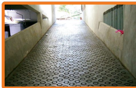
'O' Ring Patterns on Ramp via Granolithic Casting.
