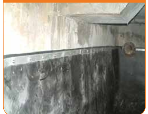
JOINING OF HDPE
