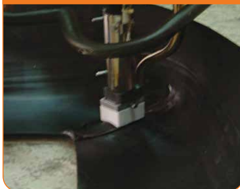
HOT AIR WELDING
